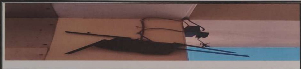
Leased line/fiber-based Wi-Fi network operating in college campus
